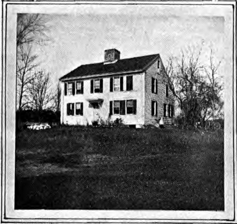
Courtesy of New Bedford Mercury.
